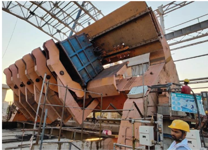
WAGON TIPPLER PACKAGE, NTPC BHEL
