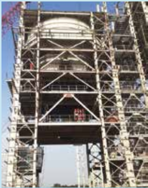
Overground bunker for Pakri Barwadih mines
