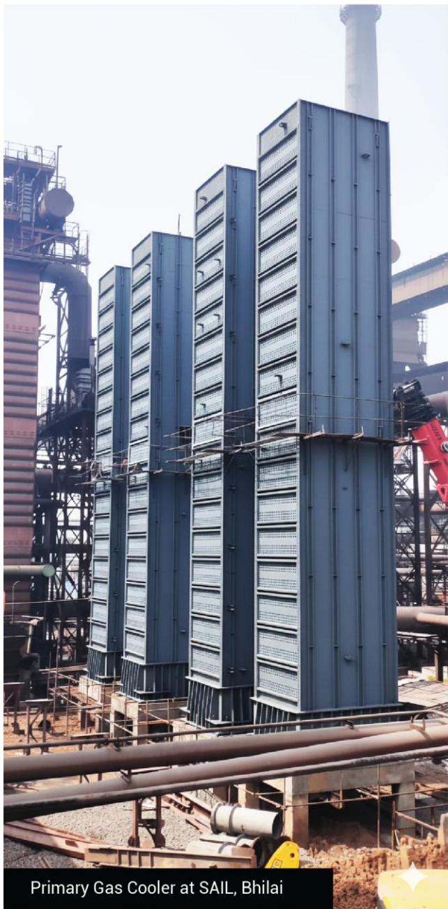
Process column at IOCL - 40m Long
